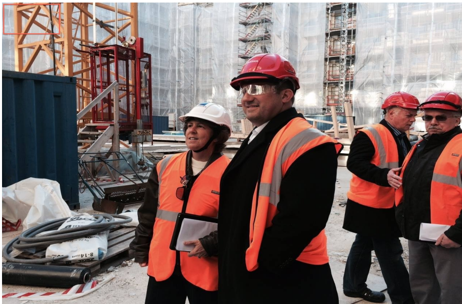
Joan Williams, CFO and Marc Vorkapich, CEO of Watercrest Senior Living Group tour the construction site of Index International AB’s residential development project, Vastermalmsterrassen in Stockholm, Sweden.
